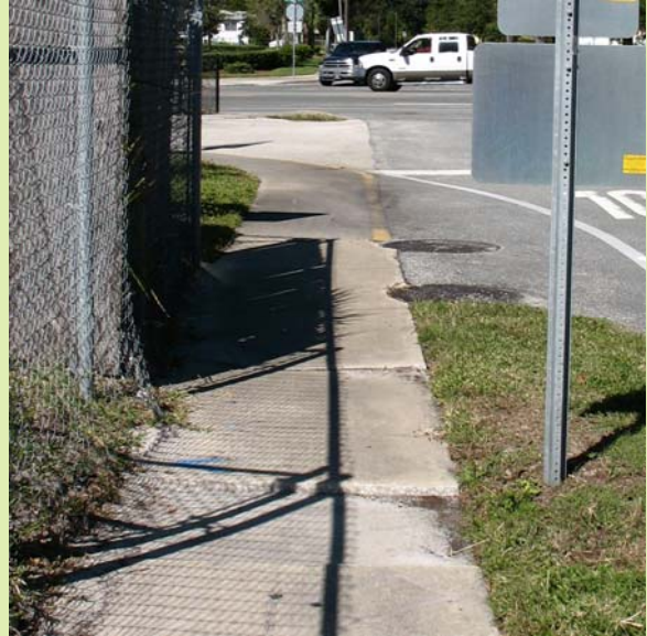
Signs are mounted too low near the sidewalk along the east side of the school
